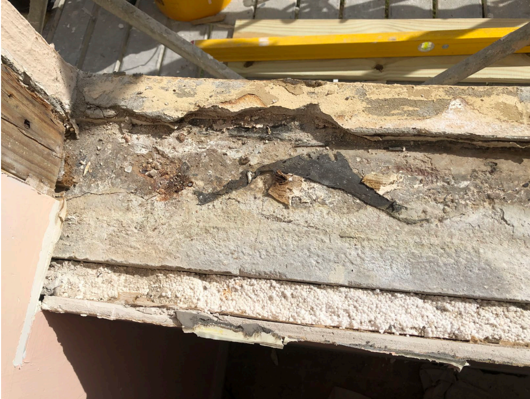
Picture 3: Cracked window sill of Unit 309
