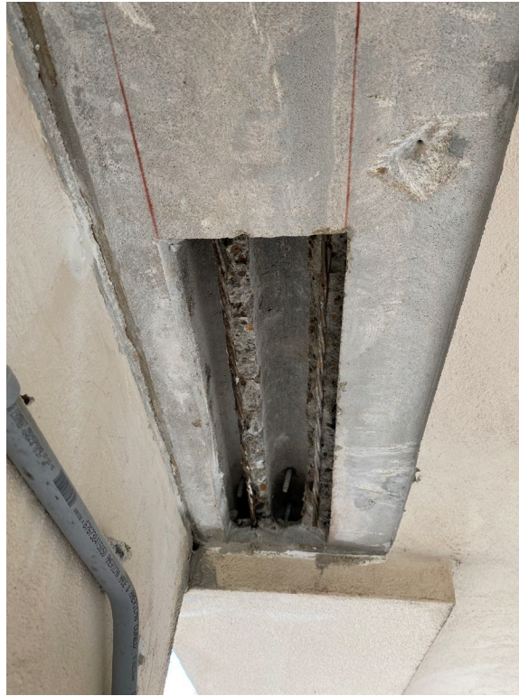
Picture 1: In-progress ceiling repair
