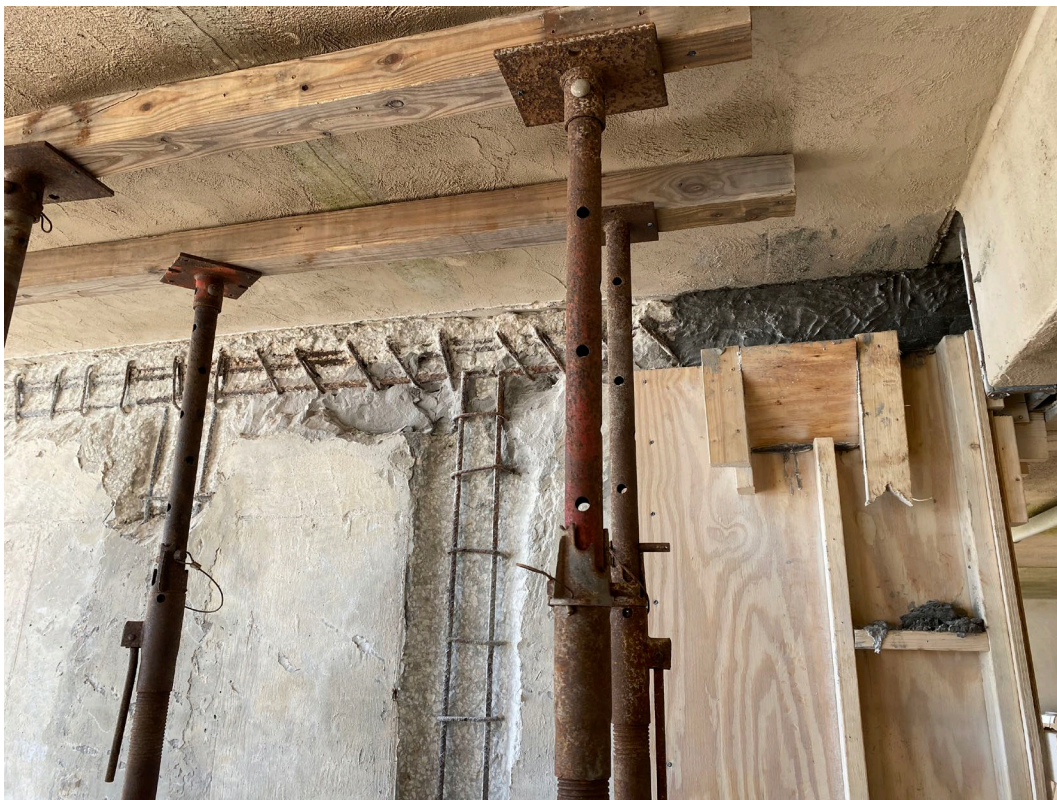
Picture 2: In-progress demon walls in parking area below the building
